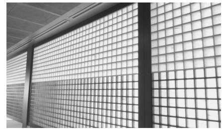
Figure 13: Shoji at courtyard
