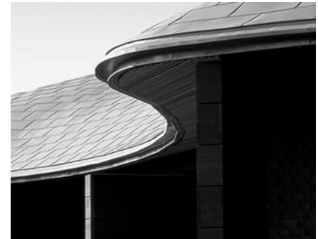
Figure 14: Titanium-plated roofs
